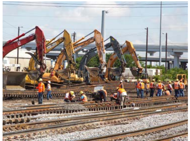
Union Pacific crews upgrade Tower 55.
