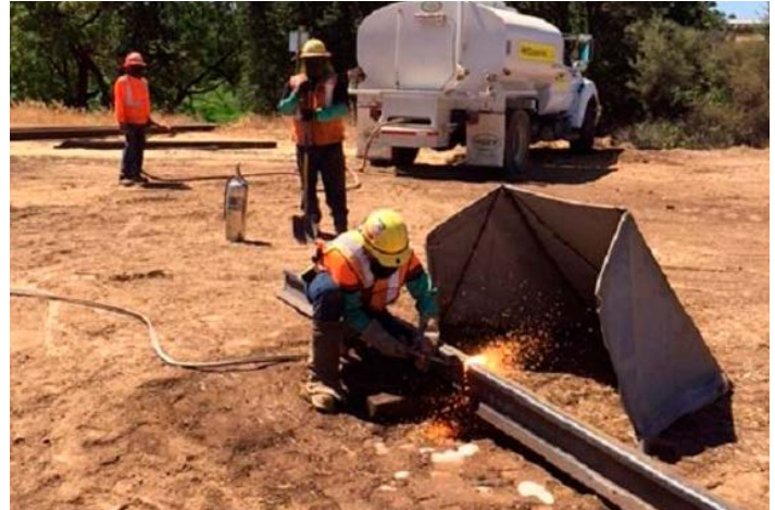
Spark shields are in place during “hot work.”
