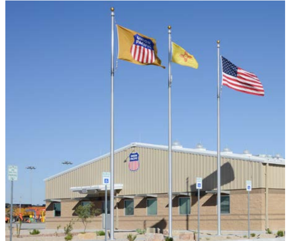
The Santa Teresa Yard Office is equipped with solar panels capable of providing 40 percent of the building's power requirements.
