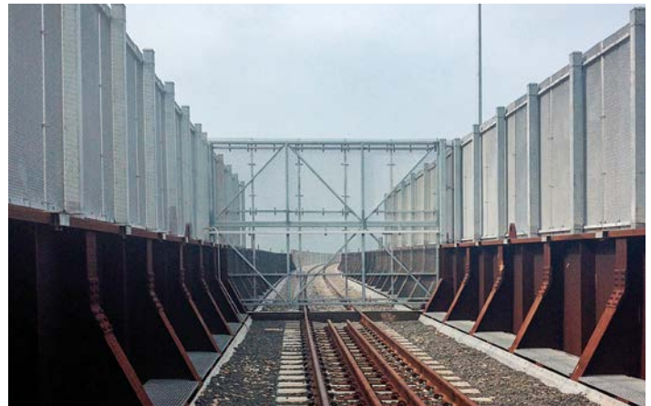
The West Rail Bridge connecting Brownsville, Texas, and Matamoros, Tamaulipas, Mexico, is the first international rail bridge built in more than a century.
