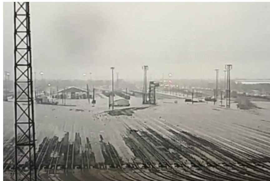
Extreme weather events, such as the devastation left by Hurricane Harvey in 2017 at Houston's Englewood Yard, make flood risk management critical.
