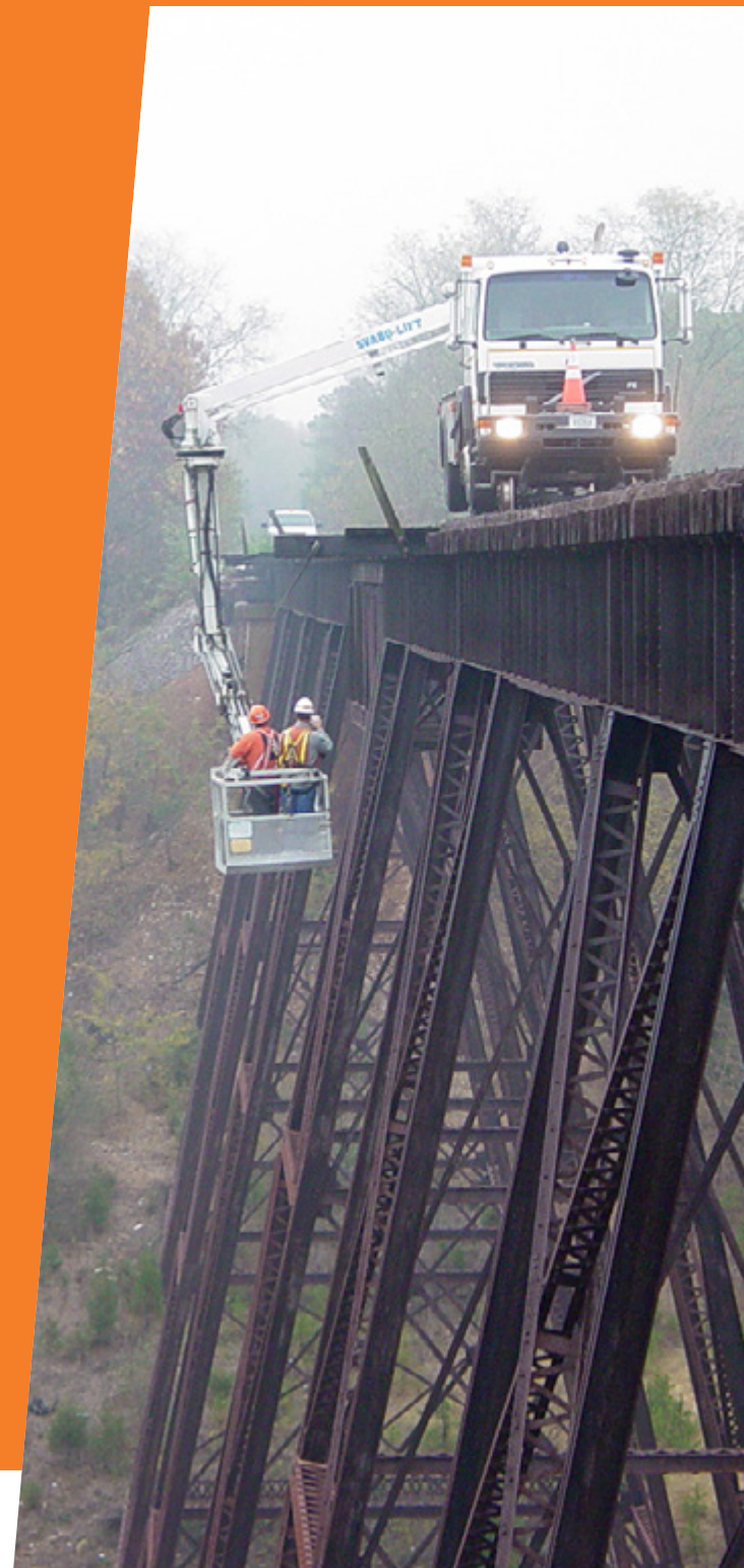
A snooper truck allows bridge inspectors to more easily and safely examine structures.
