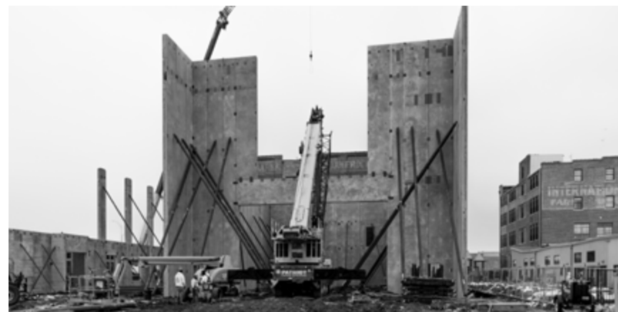
Construction begins on the Polina and Bob Schlott Performing Arts Center.
